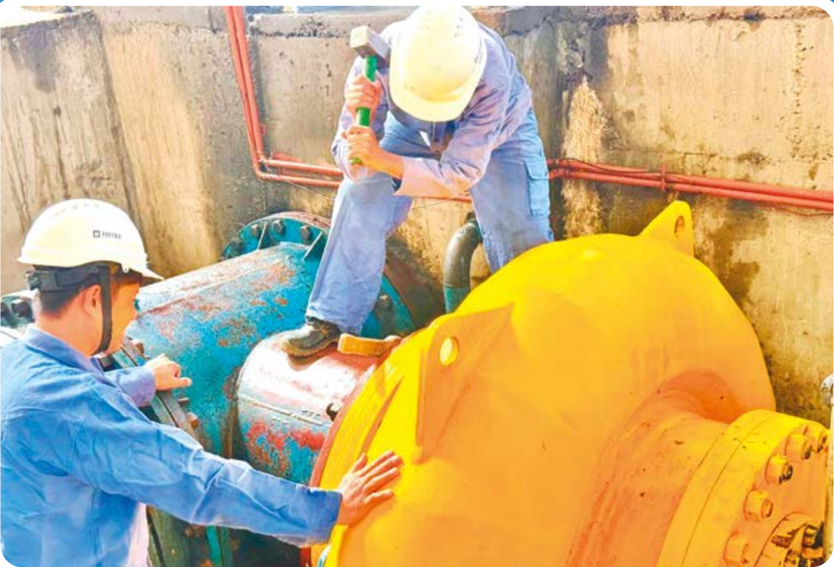
PRV Installation
